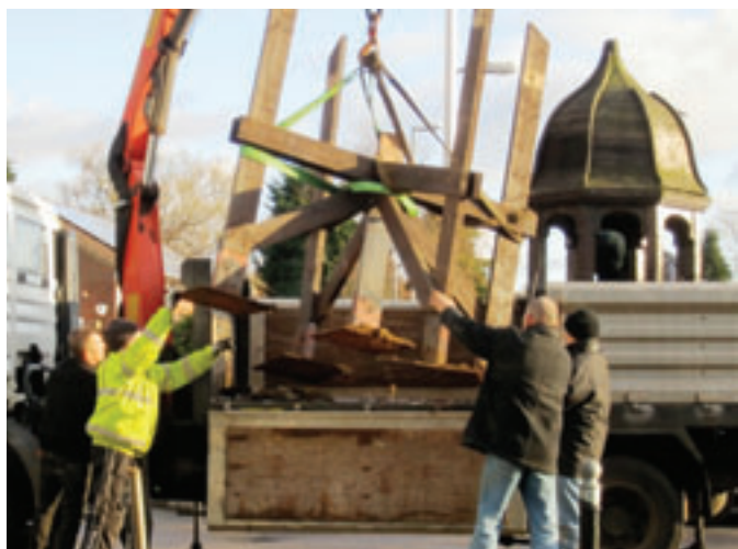
Claytons bell on the move to its new home
