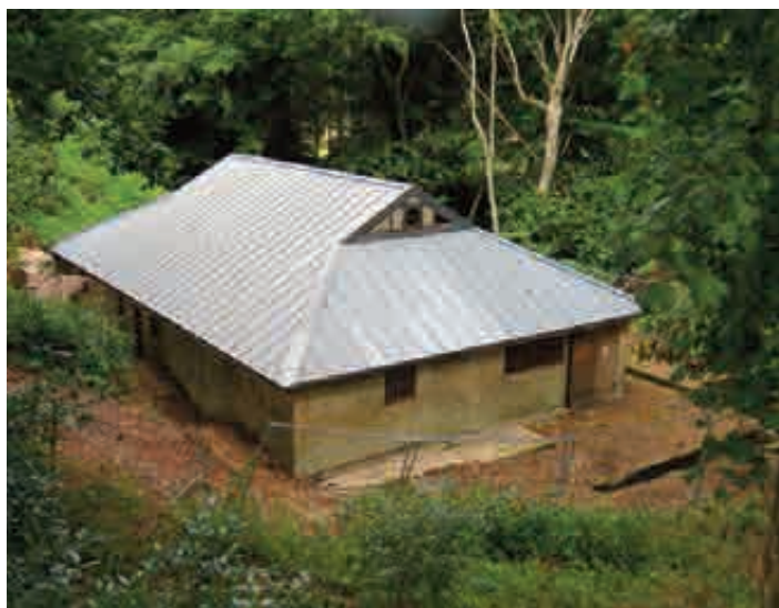
Cliveden's Generator House was almost a ruin when its structure was restored and it was roofed to keep it dry. Its machinery was removed and sent abroad when the property eventually switched to mains electricity. There are plans for its future use in the next stage of the restoration project.
